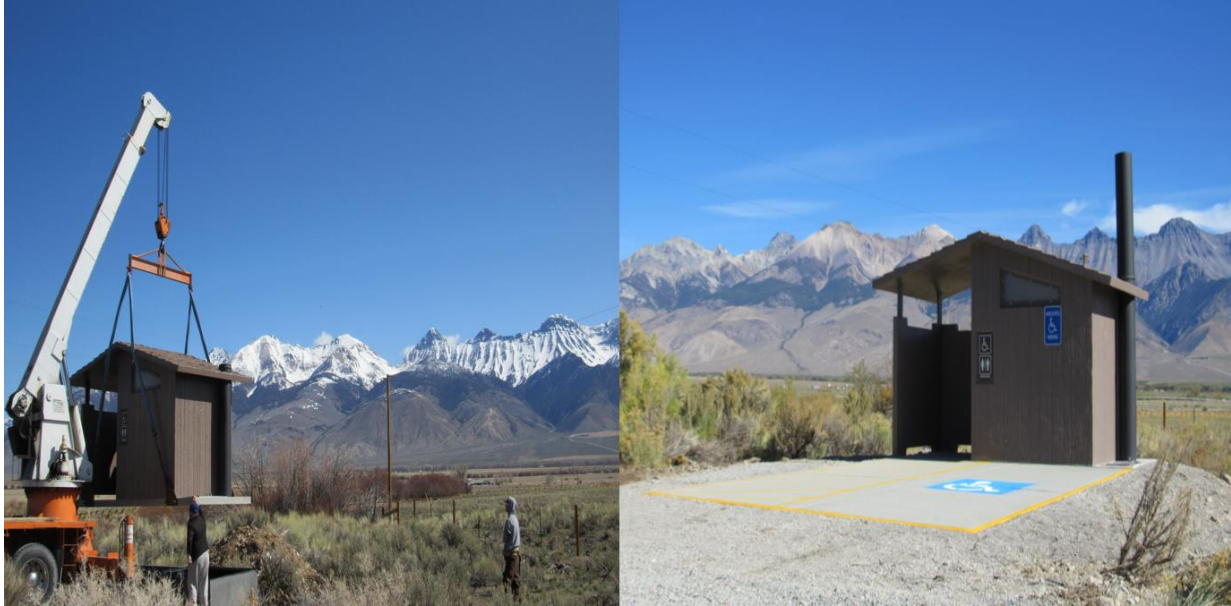
Figure 121. Installing a vault toilet at Mackay Fish Hatchery.
