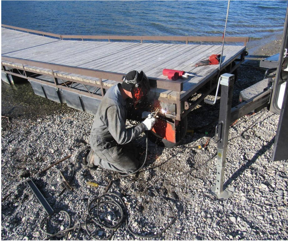
Figure 122. Repairing a section of dock at Mackay Reservoir's upper access site.
