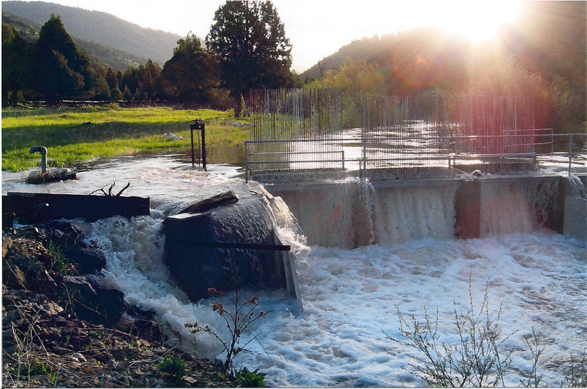
Figure 46. High water at the Rainey Creek weir on May 19.
